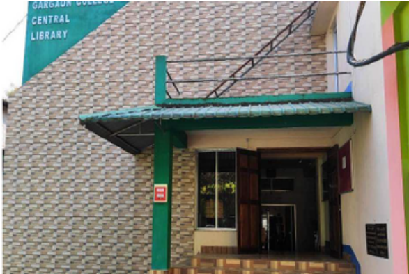
Front View of the Libraray
