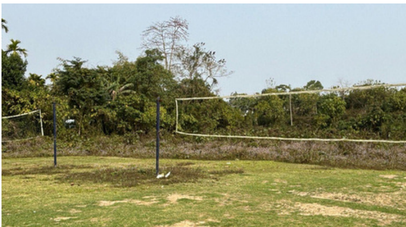
Photo 3: Volleyball Court under construction
